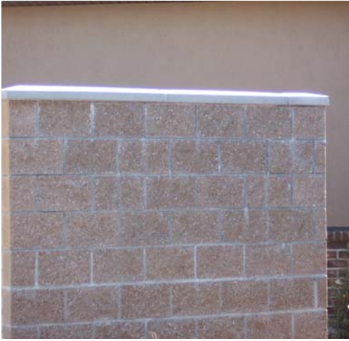
Permitted – Finished CMU
