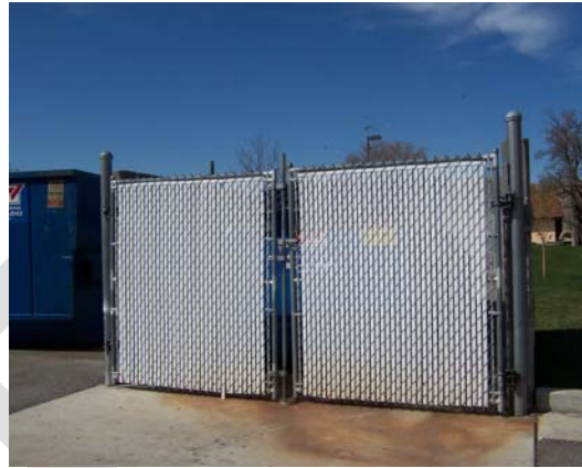
Prohibited – Chain link
