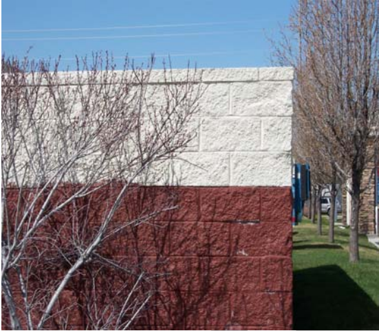
Permitted – Painted finished CMU
