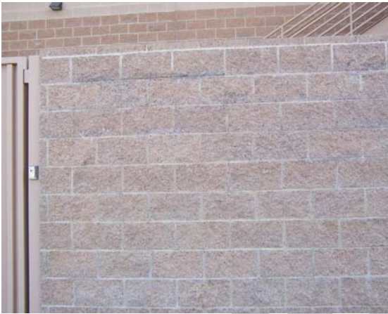
Permitted – Finished CMU
