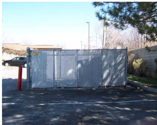
Prohibited – Chain link
