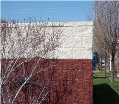
Permitted – Painted finished CMU
