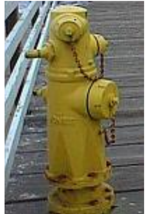
Wet Barrel Hydrant
