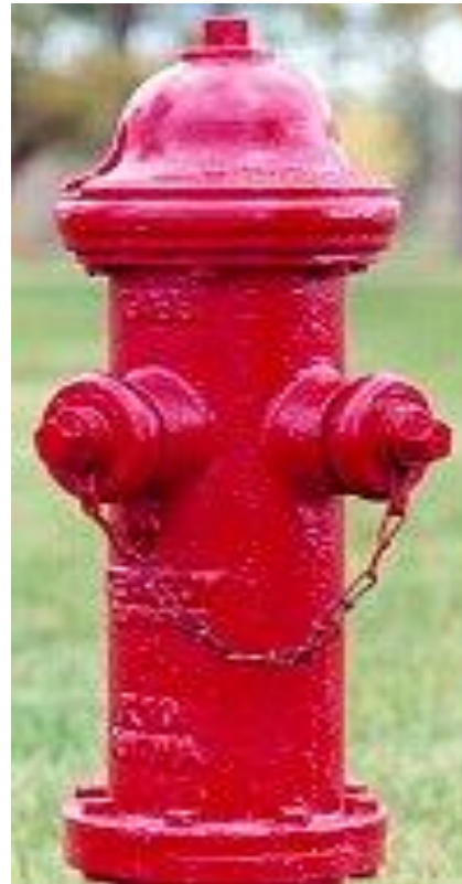
Dry Barrel Hydrant
